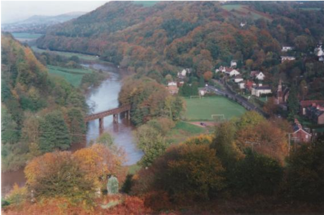
Lower Redbrook Village - Railway bridge which carried the Wye Valley Railway until 1959, linking Redbrook Station (right bank in England), with Penallt (left bank in Wales), the sites of which are 200metres apart, but hidden in trees.
