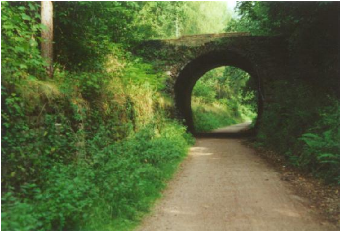
Trafalgar Arch, near Brierley - Bridge over the former Severn and Wye Railway. The bridge carried colliery 'traffic' and renovated when the former railway track was incorporated into a family cycleway.
