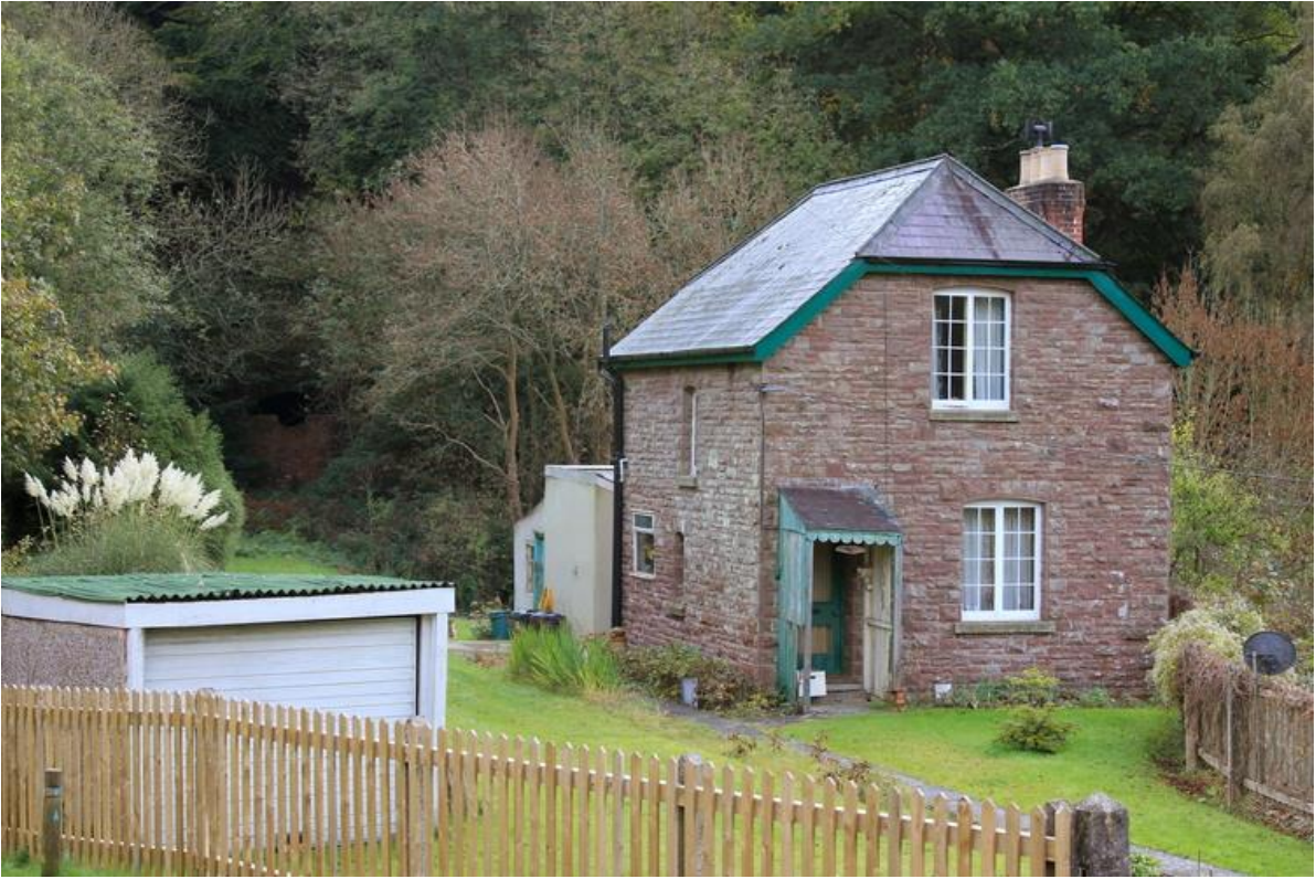
Crossing Keepers House (2010)
