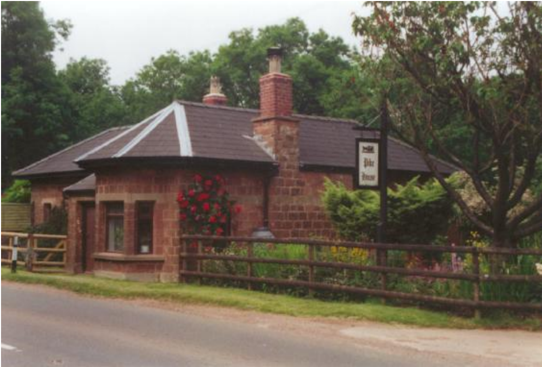
Pike House, Sling - A toll house on the Coleford to Lydney road which was turnpiked in 1795. Newland Parish
