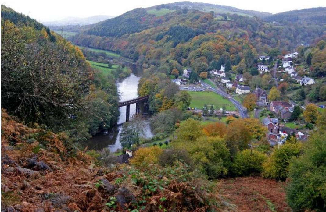
Lower Redbrook and the railway bridge show little change. New developments have taken place around the site of the tinplate works to the right of the view.
