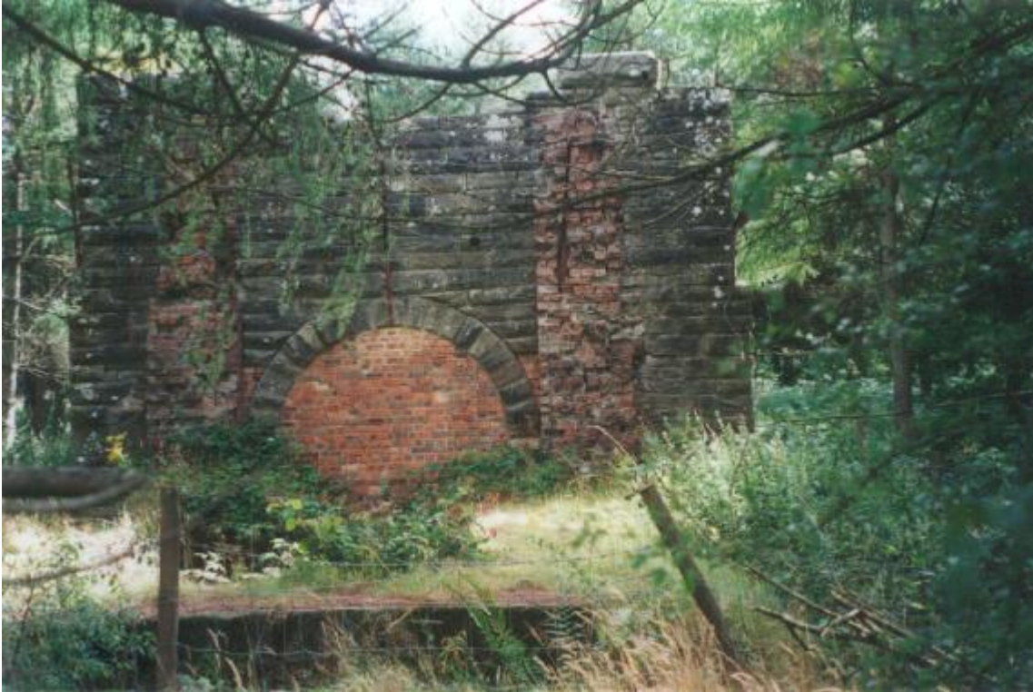
Fairplay engine house - Iron mine engine house near Plump Hill. Cinderford Parish
