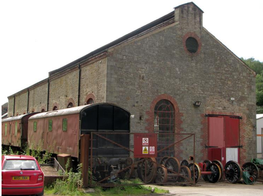
The building shows some minor modifications but the large side windows are mostly obscured by the rolling stock. The presence of this and the wheels and axles reflect the continuing success of the workshops.
